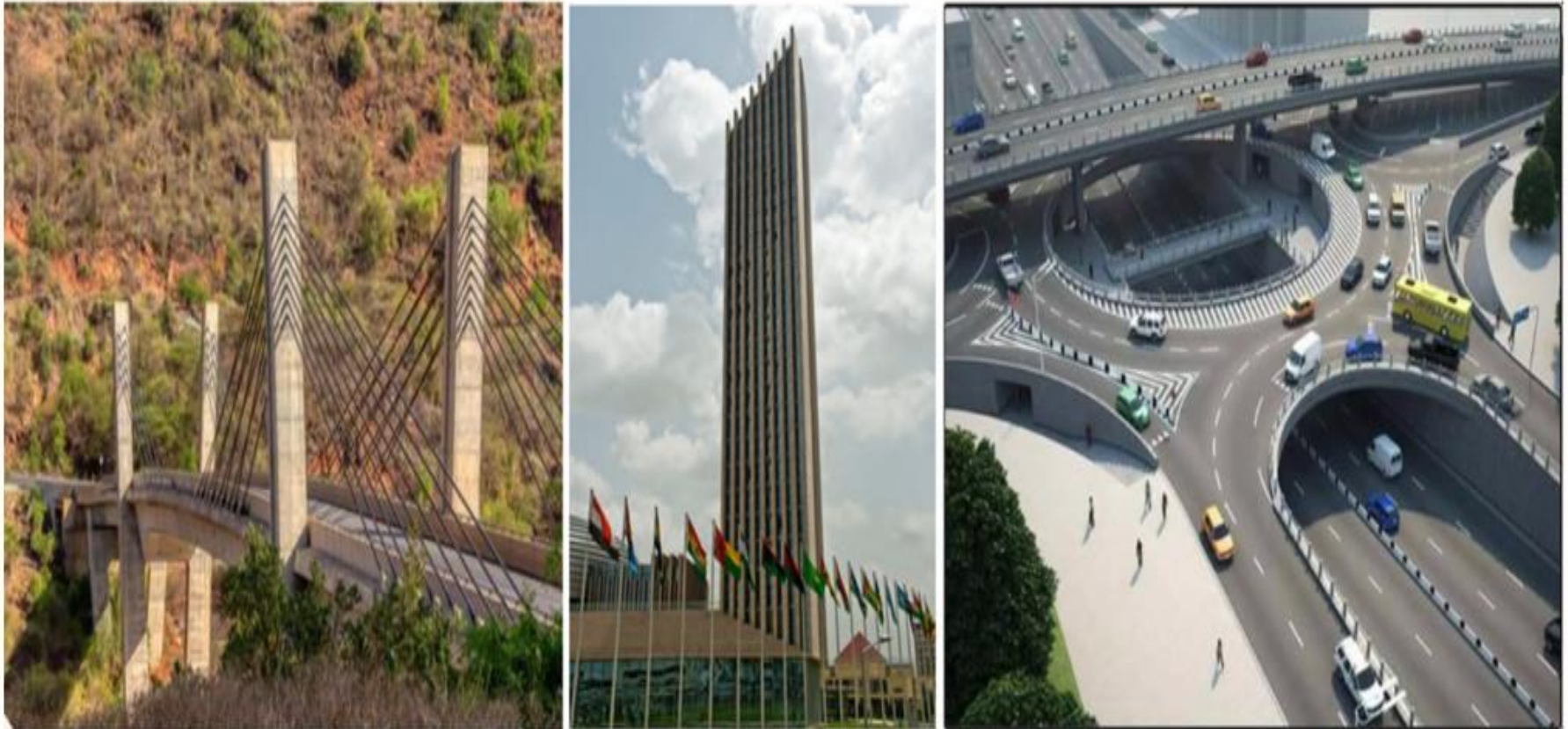
Figure 1.7 Civil Engineering in (a) Suspension Bridge (Hedase Bridge) (b) Building construction (Africa Union Head Quarter, Addis Ababa) (c) Transportation Engineering (Gotera interchange road)
